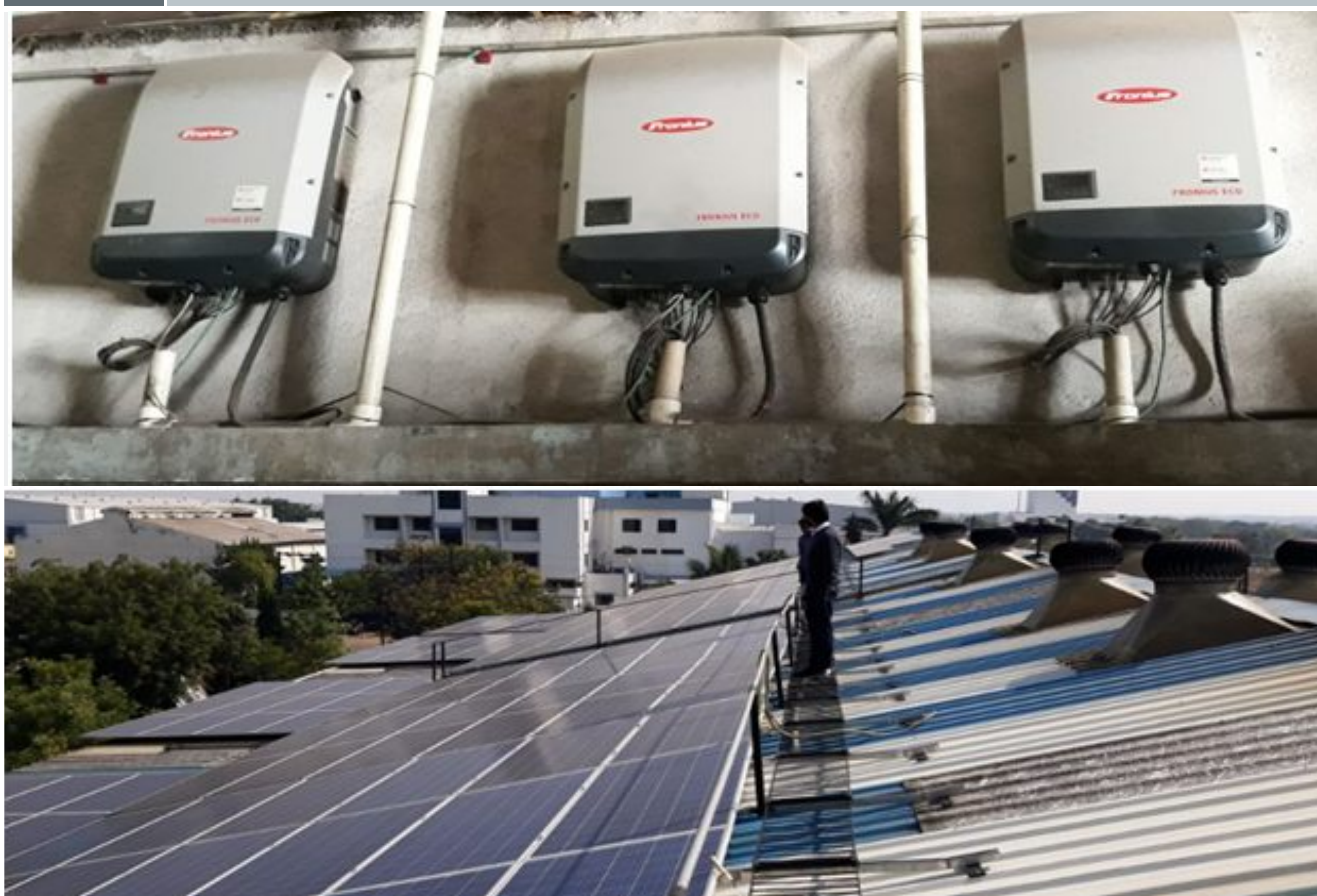
Figure 19 Inverter installation and rooftop solar project
