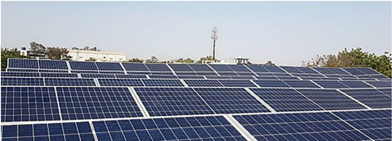
Figure 10 42 KW rooftop solar at of M/s Ashapura Industries
