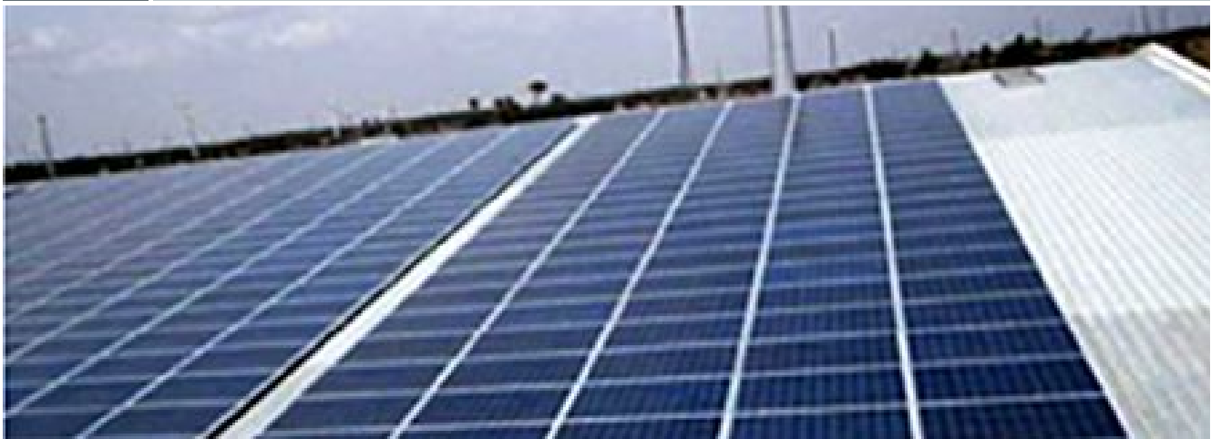
Figure 12 1 MW Rooftop solar plant at SRG apparel
