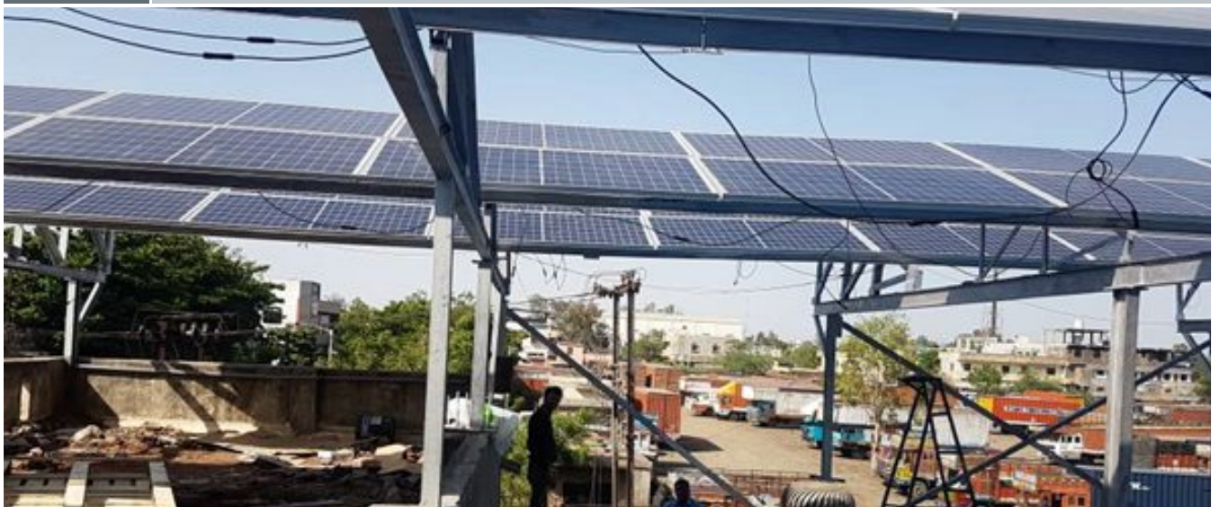
Figure 24 Superstructure at 40 kW project to achieve shadow free south side and better generation
