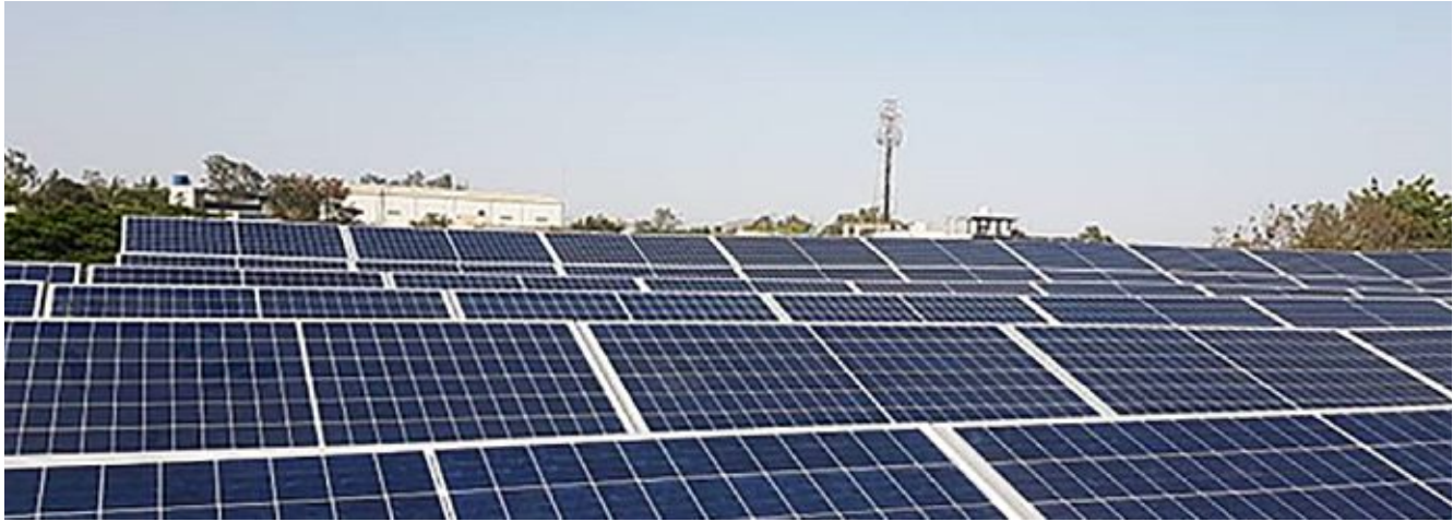
Figure 21 Rooftop solar project at AEPL unit at Waluj, Aurangabad
