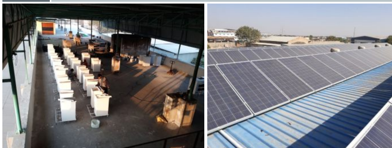
Figure 14 Solar rooftop at a handicrafts unit, Jodhpur
