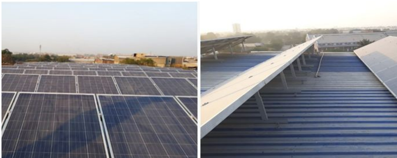
Figure 34 66 KW rooftop solar project at Sharma industries Unit 3 - Jodhpur
