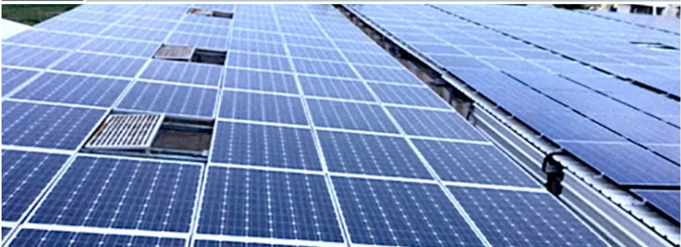
Figure 13 95 KW rooftop solar project at Hi-life Labels
